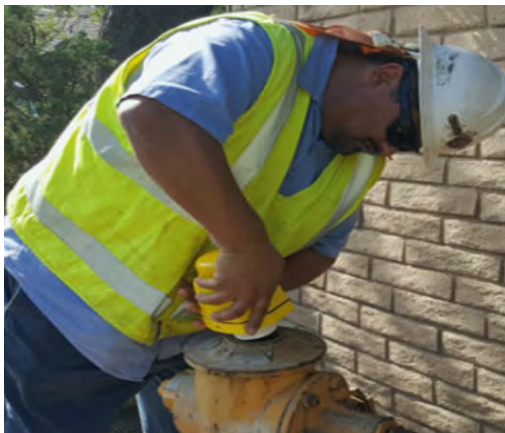
Installation of a Pressure Logger
